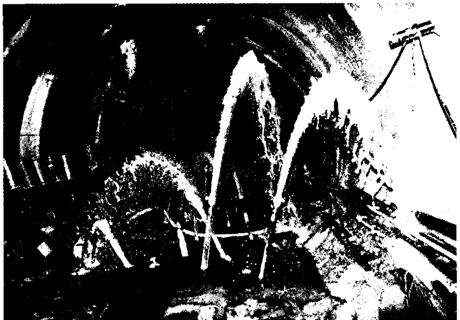
▼ 3 kilometres into the Jura mountains, LEP tunnelling was temporarily stopped by an inrush of water from behind the rock face.
